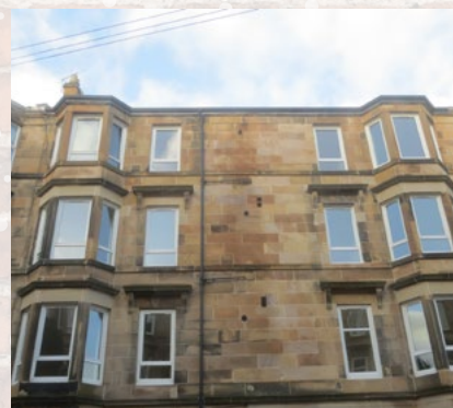
Front elevation following stonework repairs and pointing
