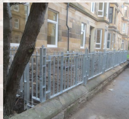
Stone cope repairs and new railings
